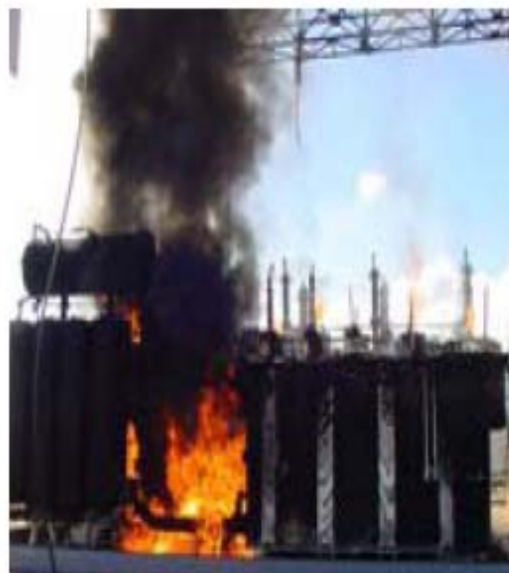
Ph. 4 Transformer fire caused by 11kV cable termination failure
