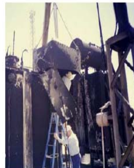
Ph 5 cable box after fire in ph.4. Cables & gland plate blasted off by arcing fault
