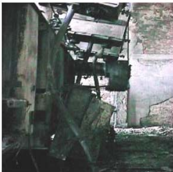
Ph. 3 Burnt out 240 MVA transformer after a 132kV cable termination failure
