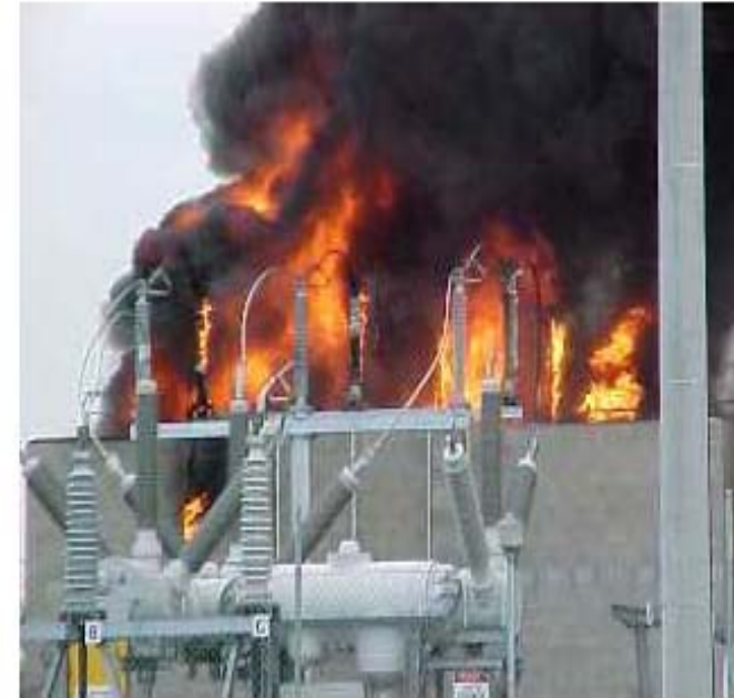
Ph 2. OIP bushing failure causes fire in transformer but fire contained by sound enclosure
