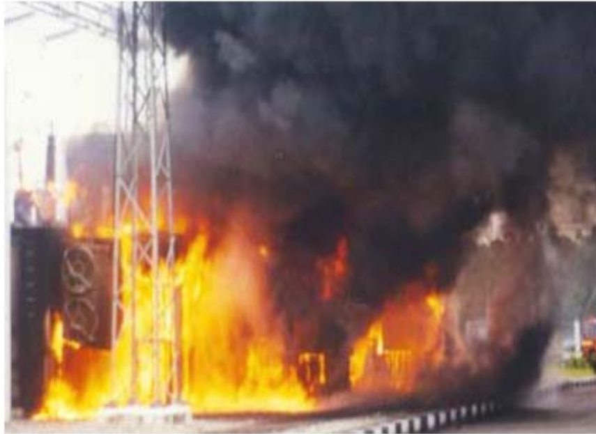
Ph 1. OIP bushing failure and oil spilling into common cable trench causes fire in two 90 MVA transformers
