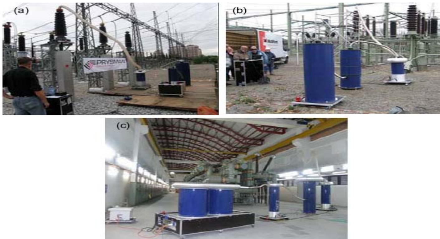
Figure 1 Examples of on-site testing and diagnosis using damped AC systems: a) after-laying testing and PD detection of a new installed 76kV/132kV XLPE power cable (19 joints/phase) with a length of 7.8km; C=1.64\mu\text{F} ; f_{\text{DAC}}=44\text{Hz} , (b) condition assessment by tan delta and PD diagnosis of a service aged 87kV/150kV external gas-pressure power cable (installed 1978) with a length of 8.5km; C=2.2\mu\text{F} ; f_{\text{DAC}}=40\text{Hz} , c) condition assessment by tan delta and PD diagnosis of a service aged 230 kV Cable oil-filled (installed 1976) (48 joints/phase) with a length of 13.3km; C=4\mu\text{F} ; f_{\text{DAC}}=29\text{Hz} .
