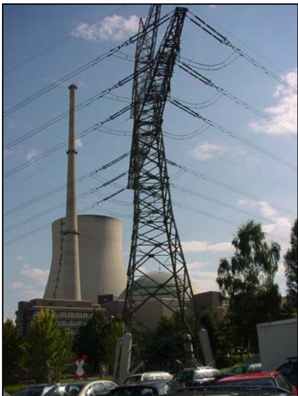
Nuclear Power Station ISAR 2 EON AG
